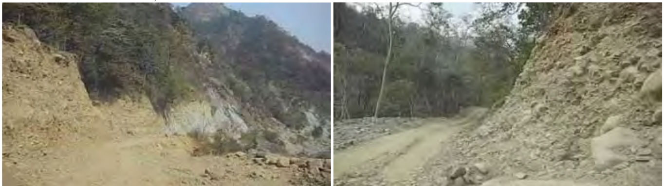
Hill side cutting in progress
