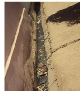
Labour Colony, Jamul. Water Pipes by Municipality pass through open sewer lines.
