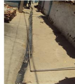
Labour Colony, Jamul. Water Pipes by Municipality pass through open sewer lines.
